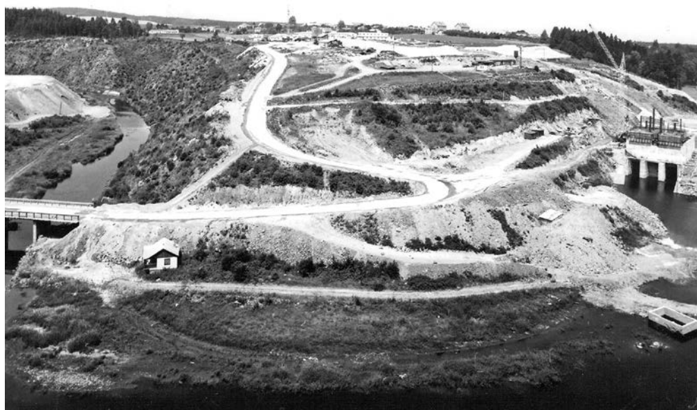
Figure 56: The Římov Reservoir – construction of the dam 1974–1975. Photo from the Archive of Vltava River Authorities.
