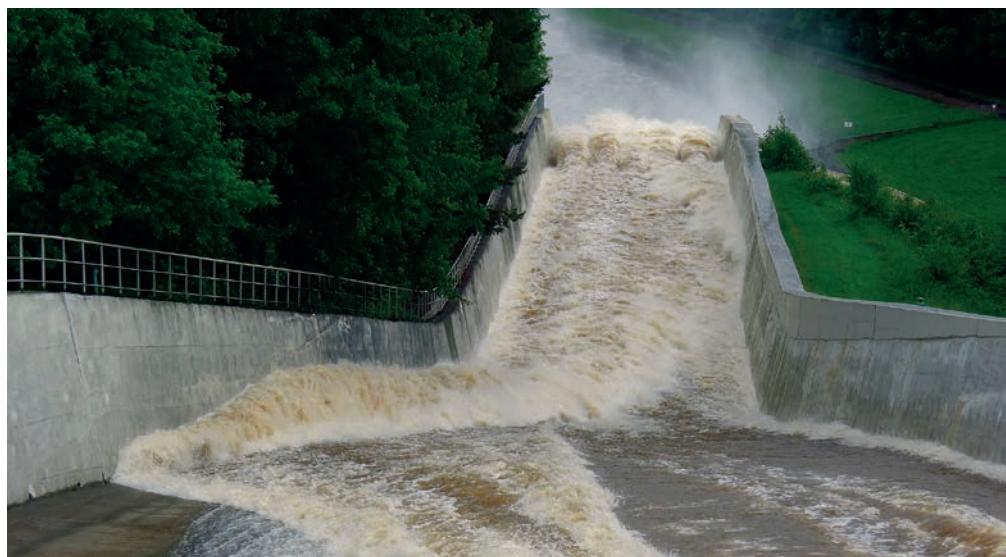
Figure 44: Water withdrawal over the spillway of the Římov Reservoir during the high inflow episode in June 2013.
